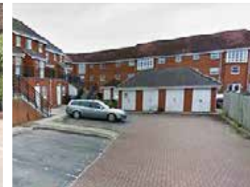
Garages create a dull façade and dead frontage
