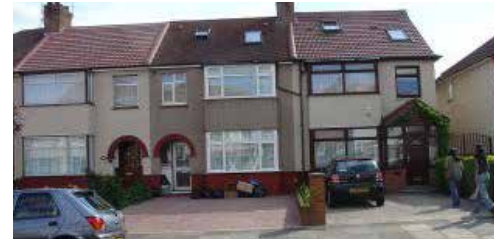
Loss of front boundaries degrades the streetscene and creates pedestrian/vehicular conflict
