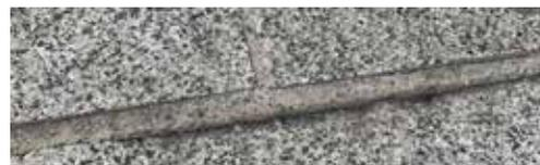
*Poor detailing and materials choice will lead to high maintenance costs. These examples illustrate spalling and cracking due to the omission of movement joints.*
